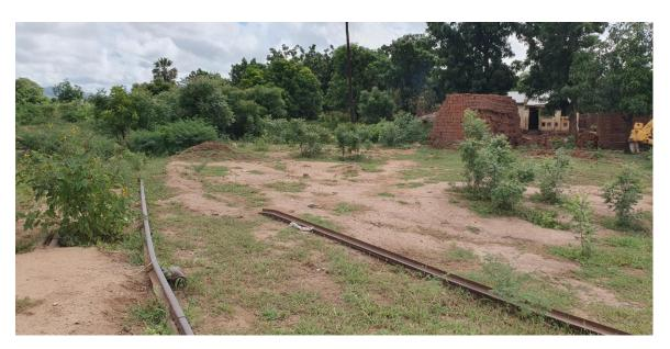
Above and Below: Around 60% of the rail sleepers on the 76km of line from the border at Marka to Bangula have been stolen, and 15% of the rail has been removed. The rail from Nsanje to the Mozambican border last ran in 1983, and from Nsanje to Bangula in 1996. The cost of rehabilitation ranges from \$750,000 per km for basic refurbishment of the permanent way, to \$3 million for more extreme reconstruction.
