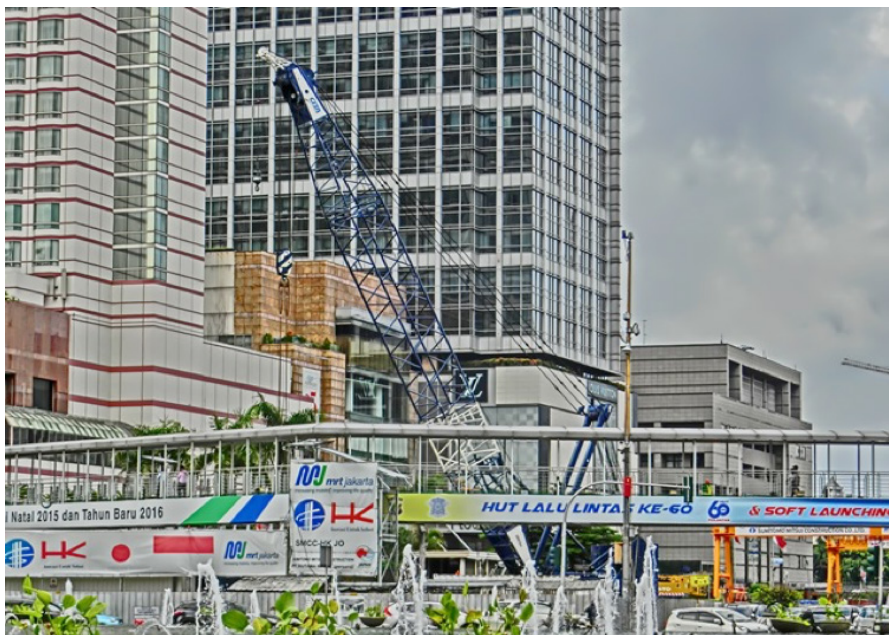
The Jalan Sudirman MRT Construction Site
